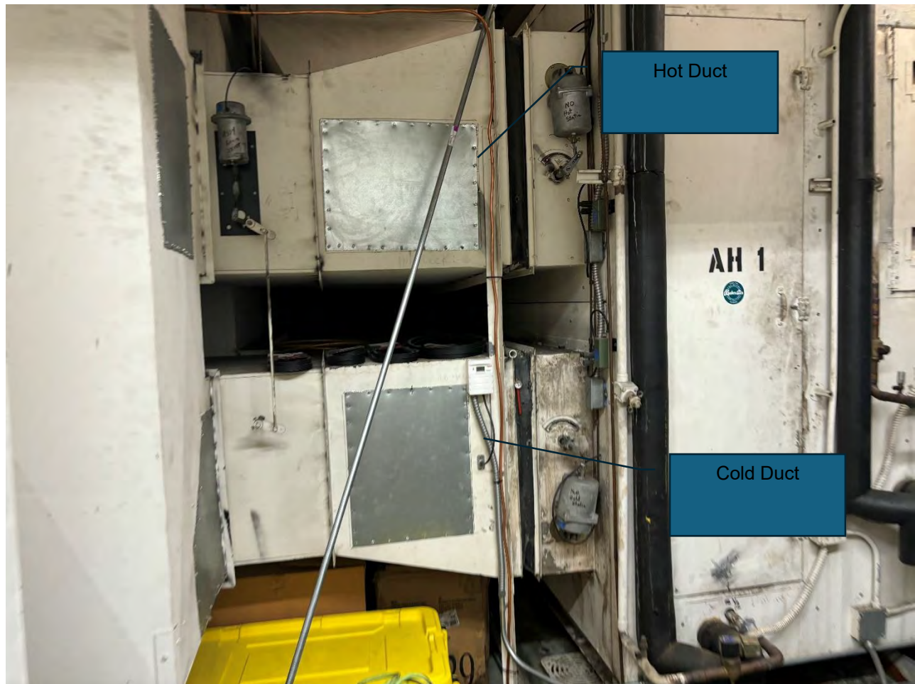
Air Handler Unit in the Mechanical Room on 2 nd floor showing double duct system.
