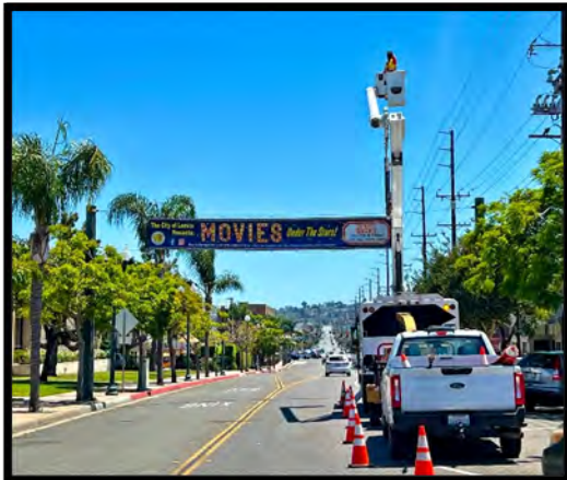
Narbonne Ave Banner Installation
