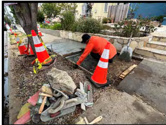
Sidewalk Panel Replacement
