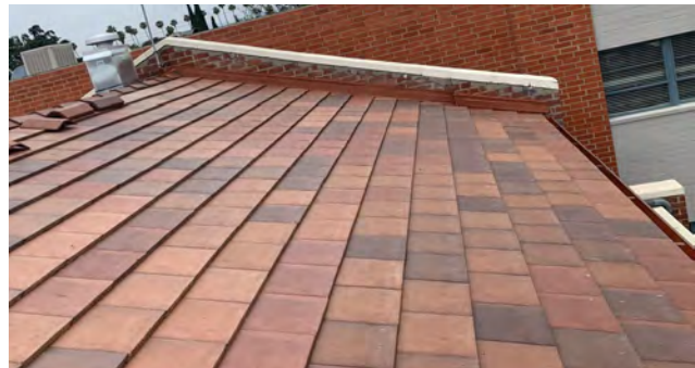
Pasadena Fire Station 33 Renovation AFTER: New replacement for roof tiles, rain gutters
