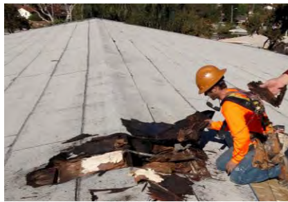
Rotted Wood Roof Framing
