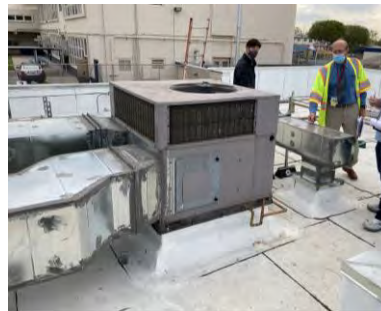
AFTER: new rigid insulation & roof, reinstall exist. HVAC equipment onto new equipment platforms.
