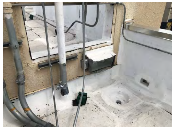
AFTER: condensate line rerouted, invasive vines removed, new coping, new scuppers
