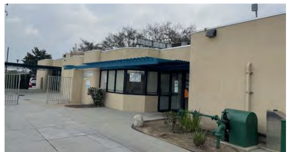
AFTER: removed invasive vines, new plaster finish-coat, painted walls.
