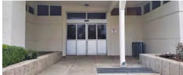
Pomona, Westmont Community Ctr. Trellis-Roof Repair Proj AFTER: new wood beam, 6x6 steel column, and new solid roof over the front entry, with scupper conductor head to direct rainwater to splash into larger catch basin.
