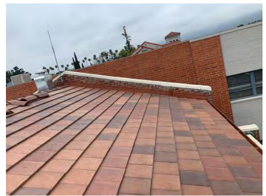
New replacement for roof tiles, rain gutters
