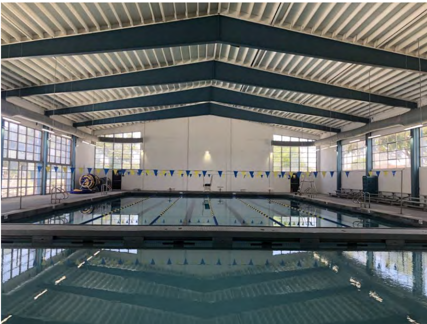
After; New Ceiling Structure, New Lighting, New Fabric Ducts
