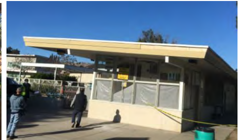
Sorensen Rec Building, Whittier, CA, In-Construction; Replace Windows/Trims, Fascia
