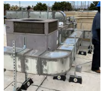
AFTER: new rigid insulation & roof, reinstall exist. HVAC equipment onto new equipment platforms.
