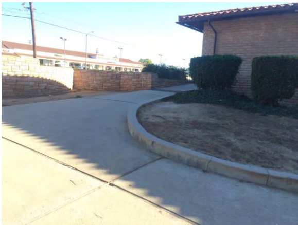
BEFORE, non-ADA compliant sloping ramp
