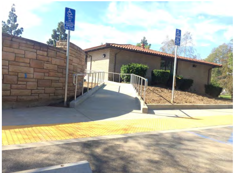
AFTER, new ADA compliant entry ramp
