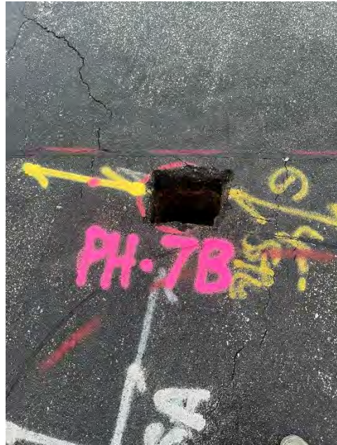
Pothole access opening
