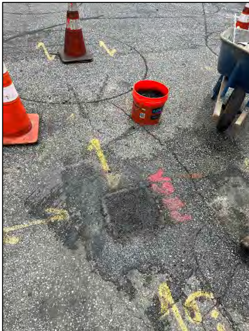
Capping of pavement following sampling
