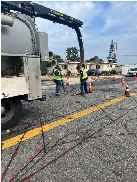
Area of pothole installation
