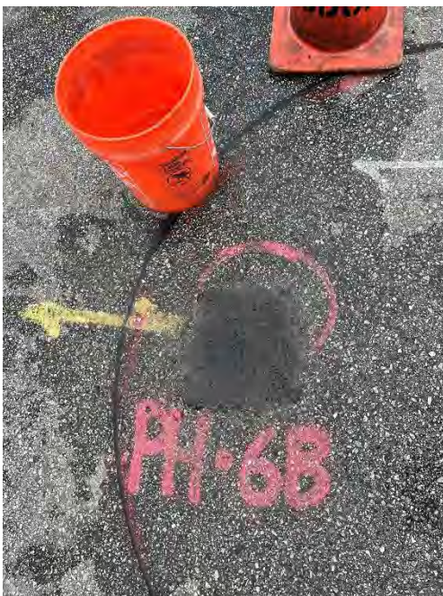
Capping of pavement following sampling
