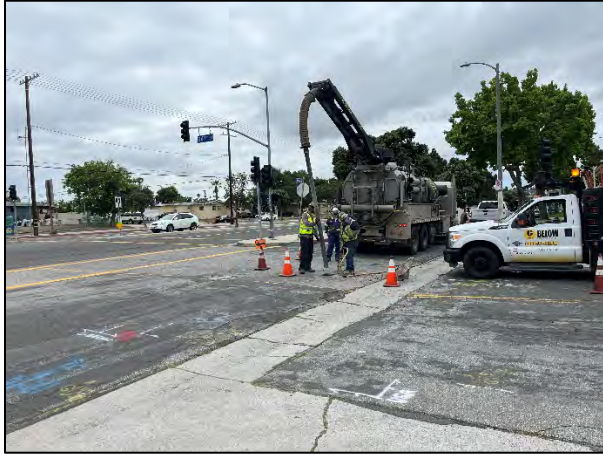
Area of pothole installation
