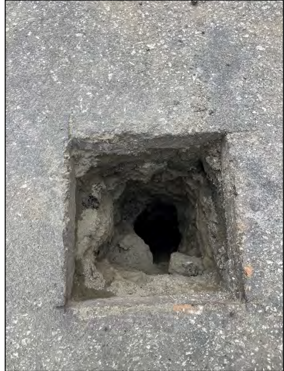
Pothole access opening - Typical
