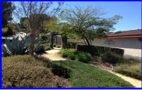
APPIAN WAY PRESSURE REDUCING STATION
