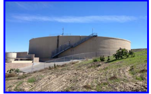
CYPRESS WATER PRODUCTION FACILITY
